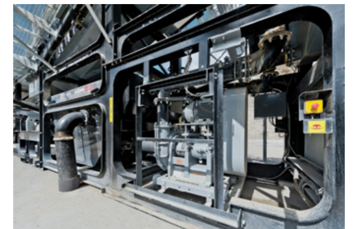
Centrifugal Pumps, Roll out for Service Access
